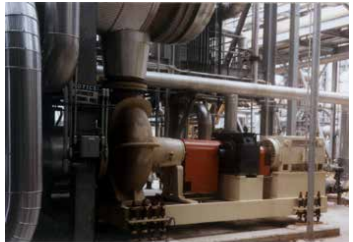
Black liquor circulation pump (3175 XL) on spring-loaded baseplate.
