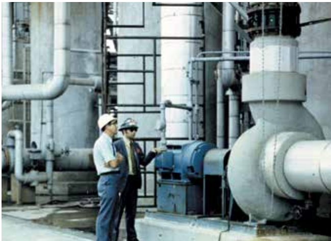
A 3175 installed in a major chemical plant.
