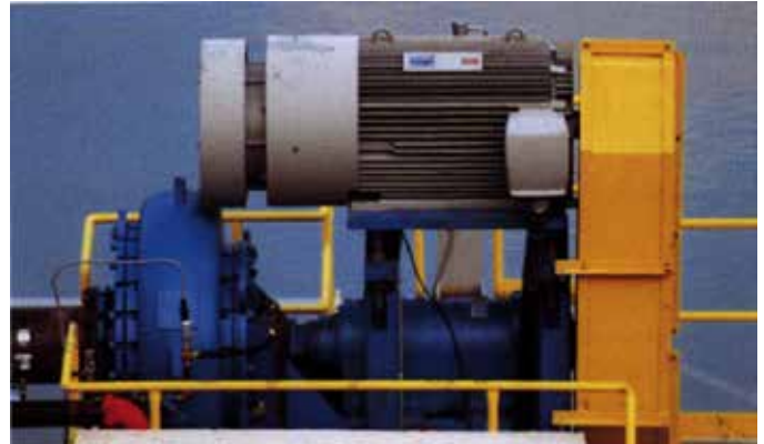
Model 5500 with 450 HP motor-mounted overhead on gold tailings reclamation service.
